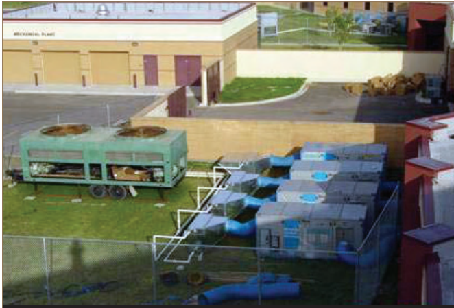
Photo 1 (left): Rental DOAS equipment at a Texas high school. Photo 2 (right) Temporary DOAS distribution ductwork.
