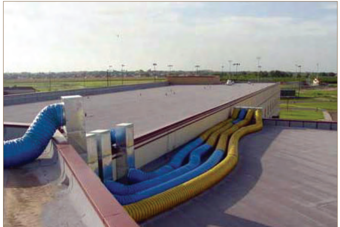
Photo 1 (left): Rental DOAS equipment at a Texas high school. Photo 2 (right) Temporary DOAS distribution ductwork.
